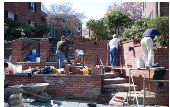
ENTRY STAIRCASE RECONSTRUCTION
