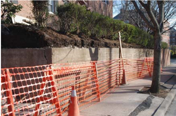
VILLAGE TREE DAMAGES SIDEWALK
