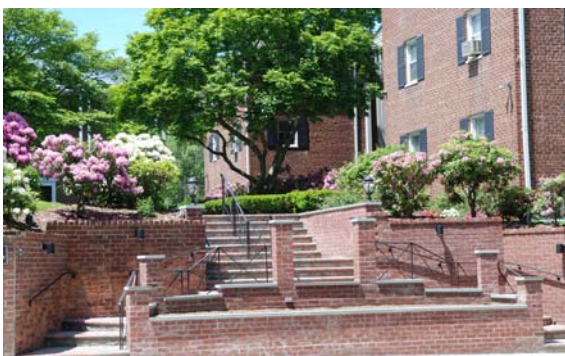
ENTRY STAIRCASE COMPLETE
